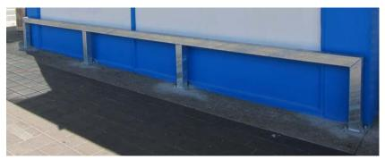
**Fixed beams** are a permanent security feature that is installed into the ground or onto the face of the building, and is intended to keep ram-raiders out. They are an excellent choice for businesses that require a high degree of security but do not require access – like shop windows.
