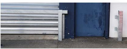
**Sliding beams** are removable by way of sliding them away to the side into brackets that are ready to hold them. They will usually be made of 89mm Square Steel tube. Special "Hamburger" type locks are fitted for added security which we fit into a steel sheath to protect them.
