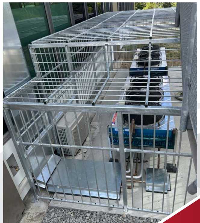
↑ Featuring a steel bar door, with double deadlocks. Locks can be according to customer requirement, like Maglock or Electronic.
